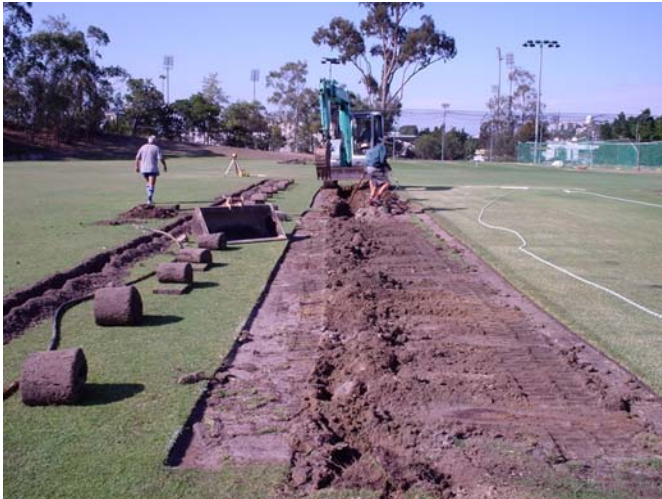
Figure 15 - Excavating wicket site
