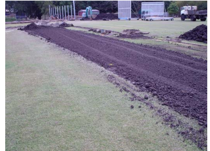
Figure 14 - Spreading of black soil
