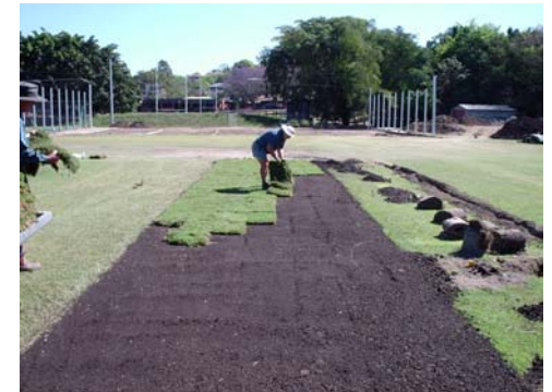
Figure 6: - Laying full turf on new wicket.
