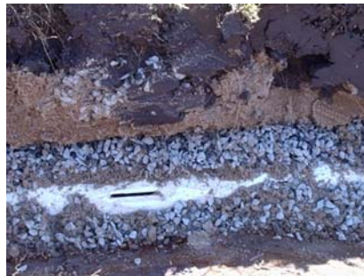
Figure 10: Drainage slotted 90ml PVC
