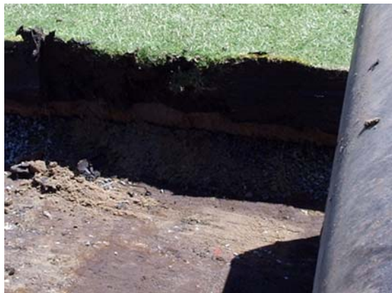
Figure 4 - Wicket depth with underlays
