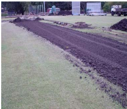
Figure 1: Spreading and levelling wicket soil
