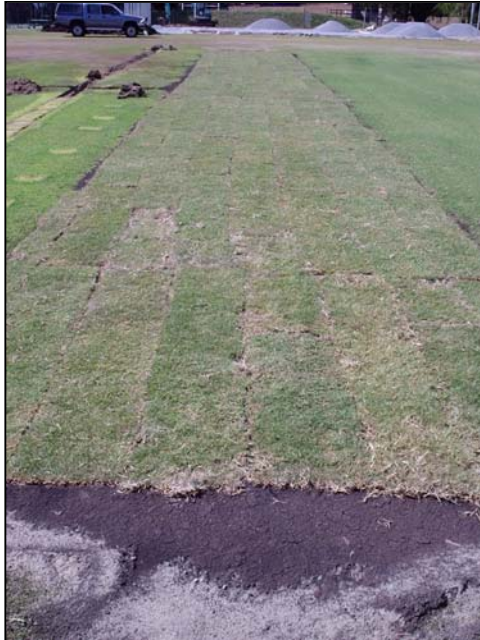
Figure 7: - Full turf laid
